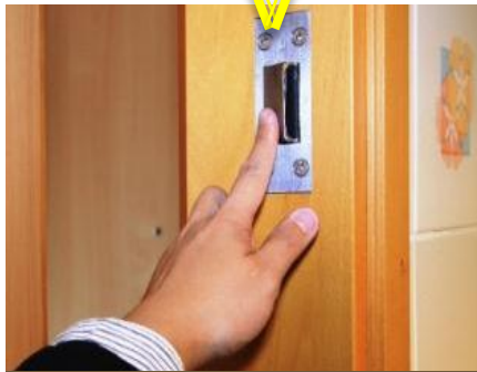
Two-way opening door - To facilitate rescue when necessary
