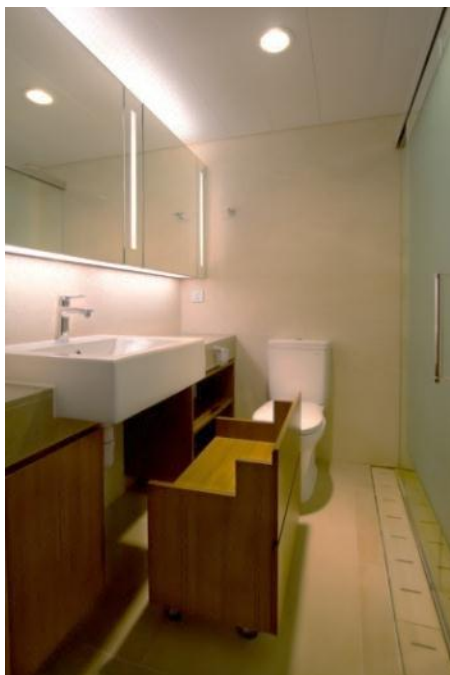
Demountable cabinet in designated bathroom
