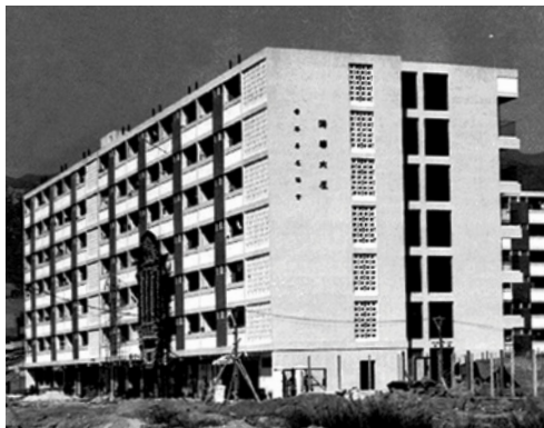
復修前 Before rehabilitation
