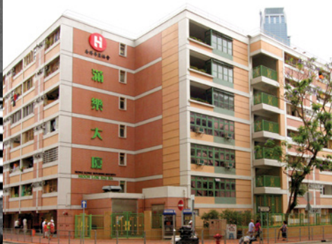
復修後 After rehabilitation
