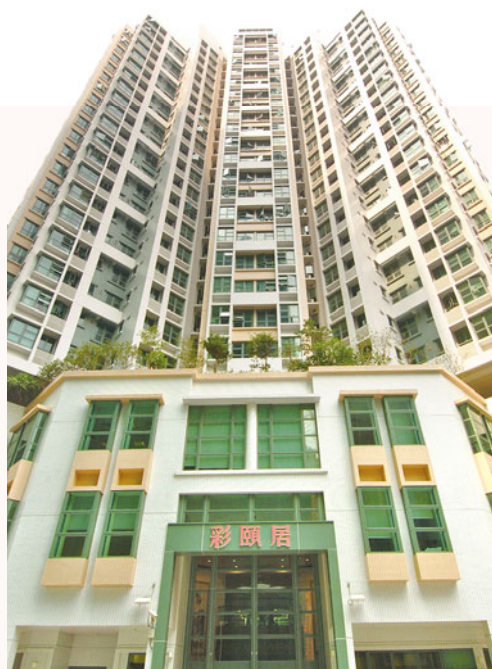
Two SEN projects, Jolly Place and Cheerful Court, enable middle-income senior citizens to age in place. 兩個「長者安居樂」屋苑樂頤居和彩頤居協助中產長者「居家安老」。
