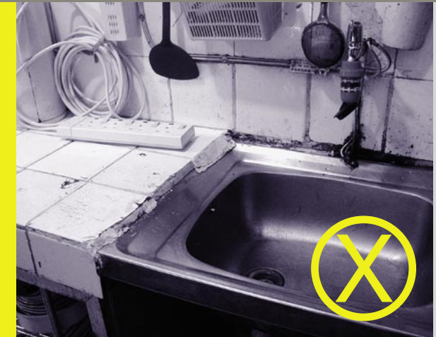
The electrical outlet is too close to the sink and water tap 電源太接近洗滌盆及水龍頭
