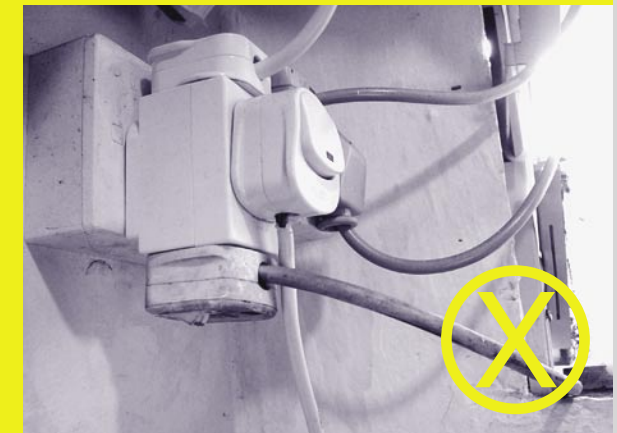
The electrical wires are overloaded 電源超出負荷
