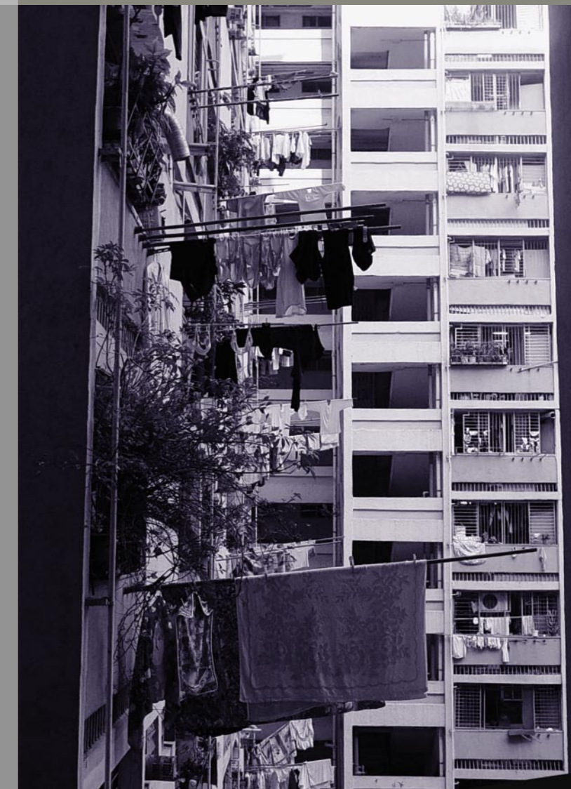
Drying racks outside the building cause nuisance and dripping water to below 露天晾衣架不但造成滋擾，亦可能向下層滴水
