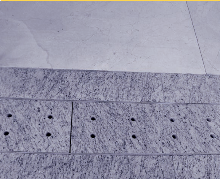
Levelled threshold at a building entrance 樓宇入口的齊平門檻
