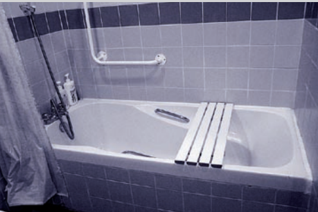
A bathtub with a bathtub board 設有浴缸板的浴缸
