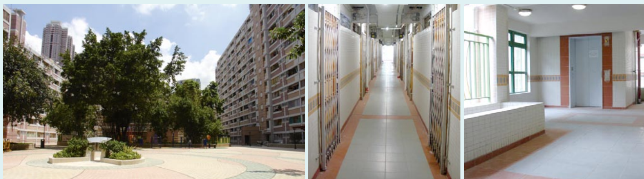
The living conditions of Moon Lok Dai Ha are greatly enhanced after rehabilitation 滿樂大廈經復修後，居住環境大為改善
