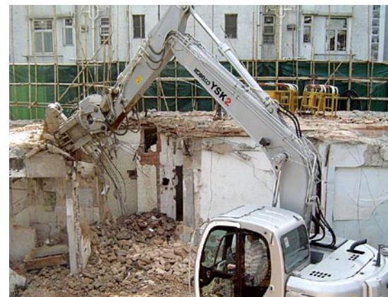
Use of hydraulic crusher at construction sites to minimise environmental impacts. 於地盤採用油壓鋼剪以減低對環境造成的影響。
