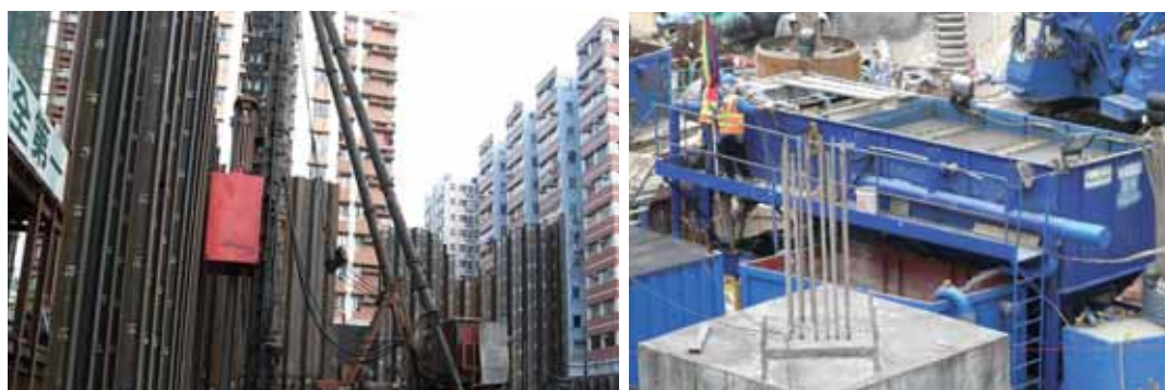
Various environmental measures: noise control (left) and waste water treatment (right) were adopted on construction sites 建築工地採用各項環保措施：減低噪音 (左)及污水處理 (右)
