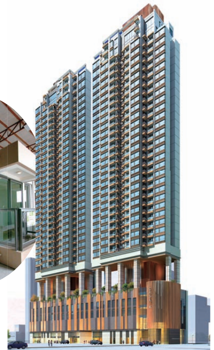
Photo illustration of the K25 redevelopment project K25 重建項目的構想圖
