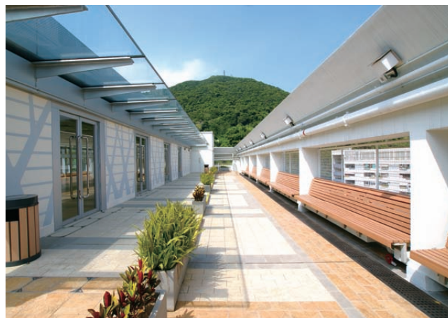
Additional leisure space was provided on the rooftop of Kwun Lung Lau after rehabilitation 復修後的觀龍樓天台增設休憩空間
