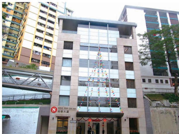
The rehabilitation of Ming Wah Dai Ha included an addition of a shuttle lift tower 明華大廈的復修工程包括新建一幢升降機大樓
