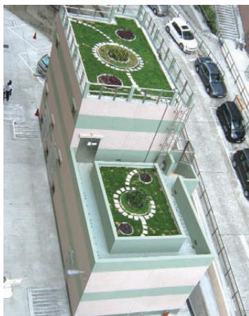
The green roof of the new transformer room at Lok Man Sun Chuen 於樂民新村新電力變壓房的綠化天台
