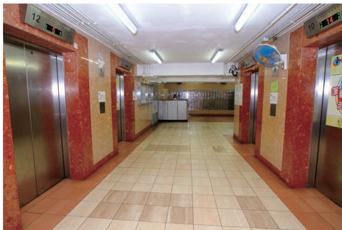
Energy-efficient lifts were installed in Kwun Tong Garden Estate 於觀塘花園大廈安裝的節能升降機
