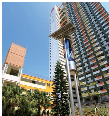
The solar energy and wind power lighting installation in Cho Yiu Chuen 於祖堯邨的太陽能及風力照明裝置
