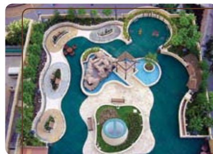
Landscaping for flat roofs to reduce solar gain 大廈天台加設花園具隔熱作用
