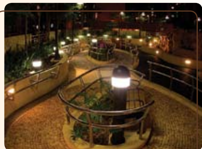
Energy-saving light fittings with timer control 備有時間掣的節能照明裝置
