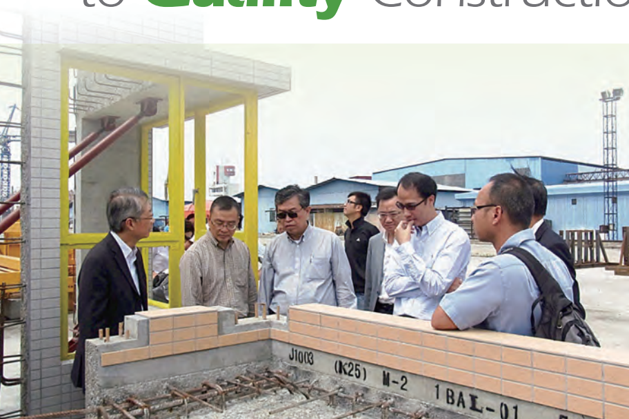
委員及同事視察東莞廠房K25項目之預製組件 Members and staff inspected the precast elements of K25 project in Dongguan
